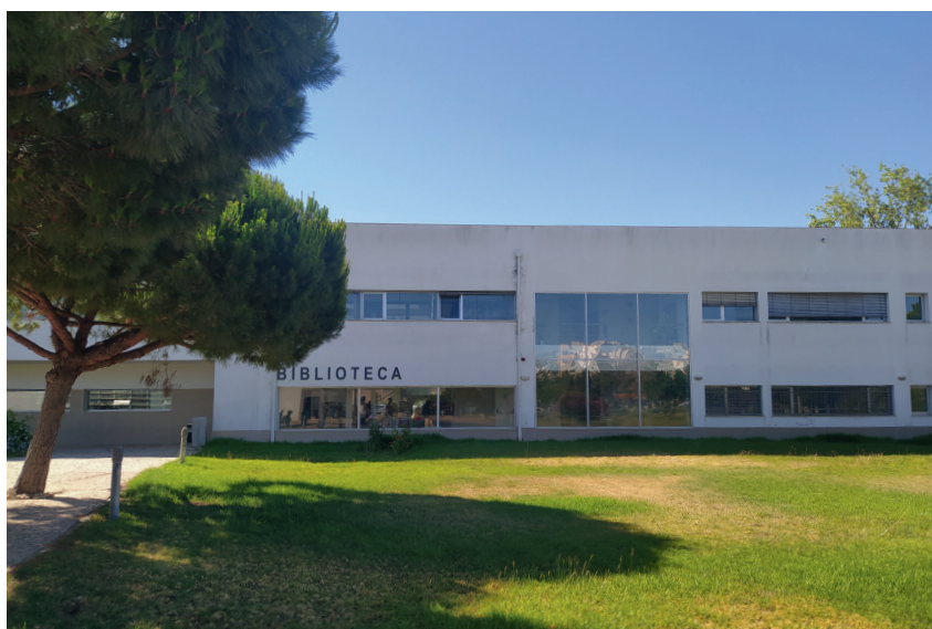
Fig. 4. Penha campus library. Photo by Ewa Kapela
